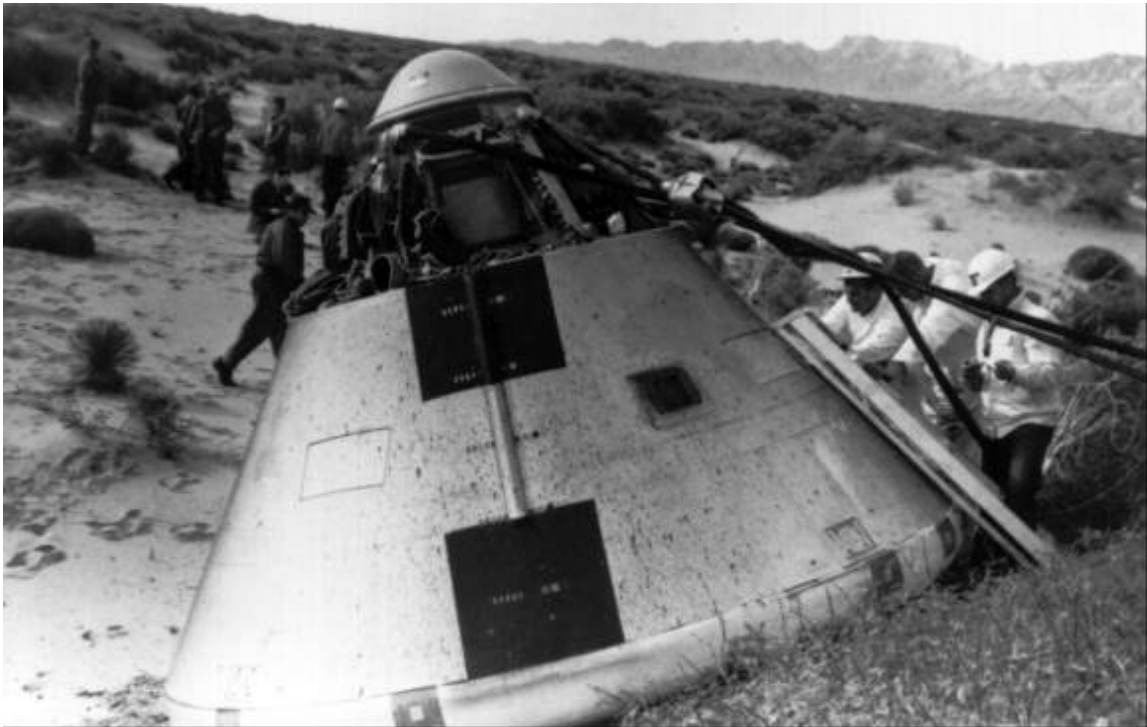
A model of the CM, below, launched by a Little Joe II in 1965, is recovered after impact on the New Mexico desert.
