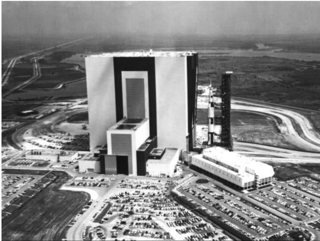
Kennedy Space Center's Vehicle Assembly Building (above; earlier called the Vertical Assembly Building) stands high on Florida's Atlantic coast; the Saturn 500-F launch vehicle rides on a mobile crawler toward the launch pad in the 1966 photo.
