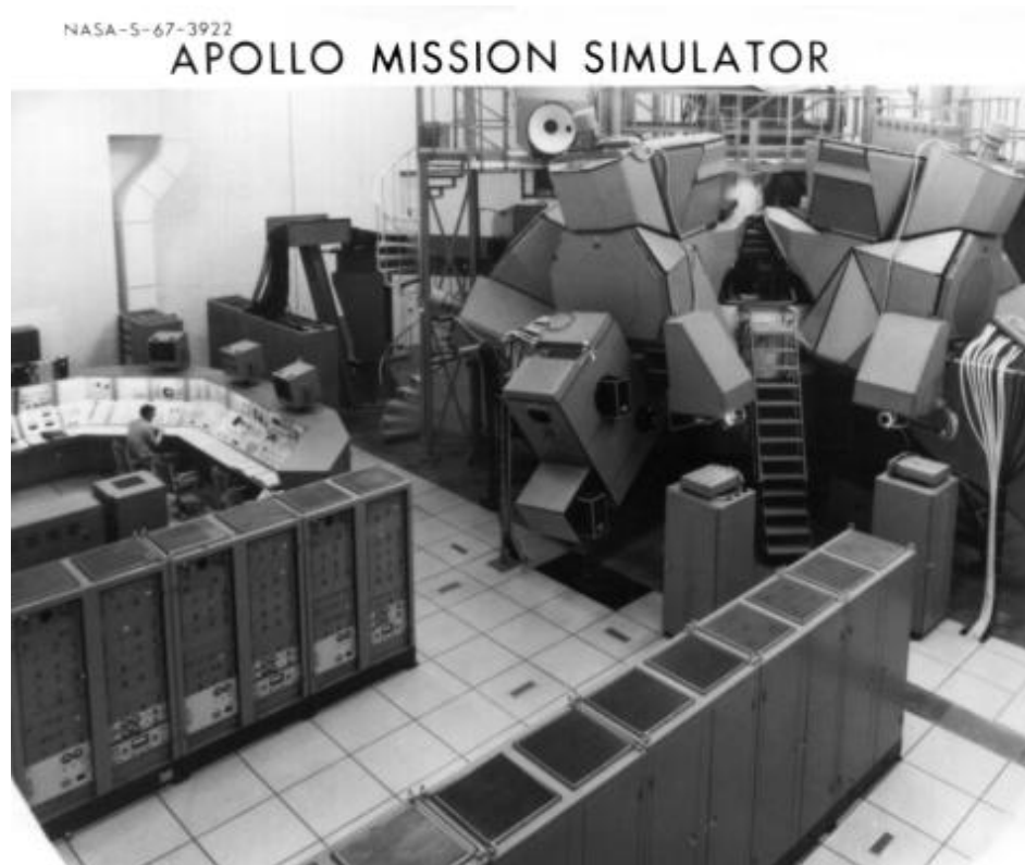
The Apollo command module mission simulator (right) at Manned Spacecraft Center, where Apollo astronauts practiced for their missions. Another simulator was at Kennedy Space Center.
