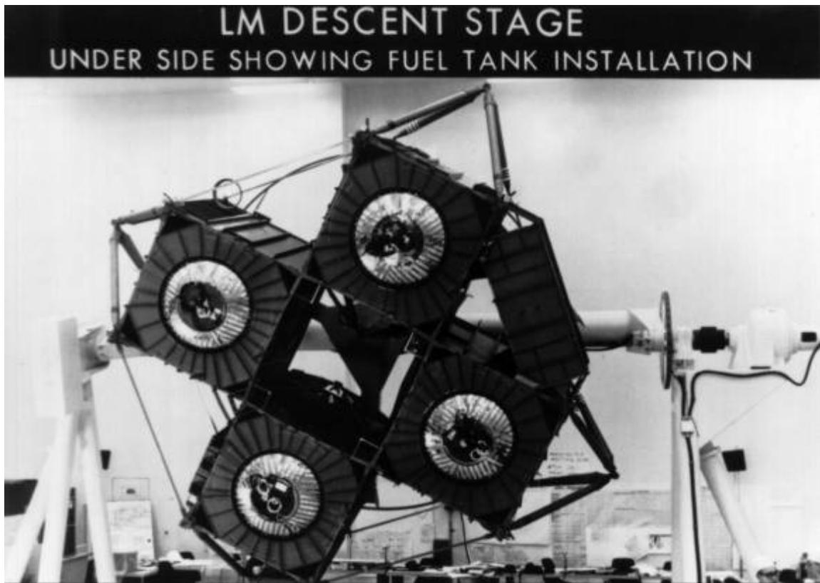
The underside of the lunar module descent stage shows fuel tank installation.
